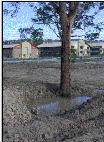
Land fill causes water to pond at the base of tree
