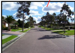
Curb and guttering
